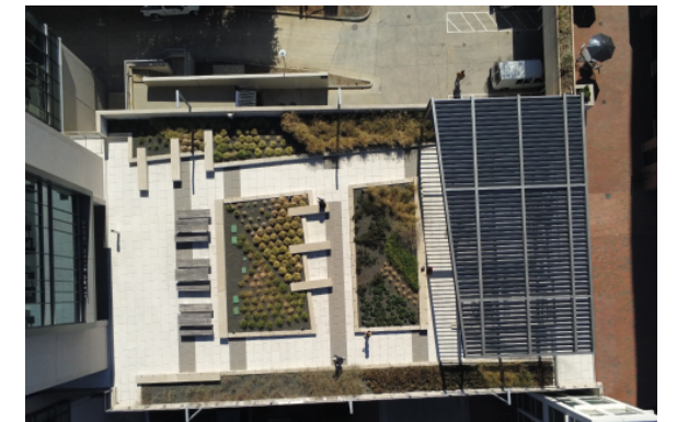
This aerial view of the LEED Gold certified Mary Ellen Jones building shows another stormwater control measure — a green roof. The area provides green space in the middle of campus (photo by CARDNL).
