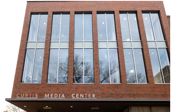
The Curtis Media Center’s rooftop PV panels can produce 34% to 87% of building energy used.
